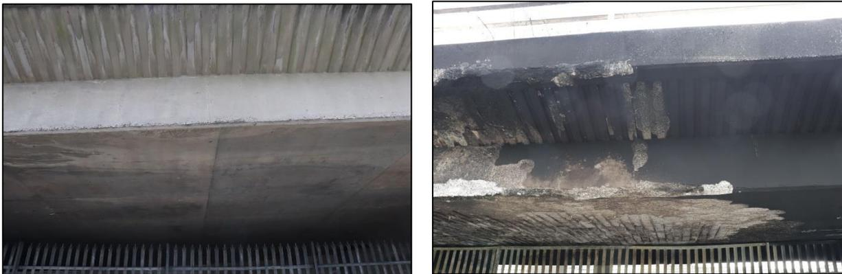
*A comparison – what the underside of the M32 should look like, compared to the fire damaged section – on the latter, the concrete has fallen away and the steel reinforcing bars are now exposed. Tests are taking place on both the concrete and the steel bars.*
