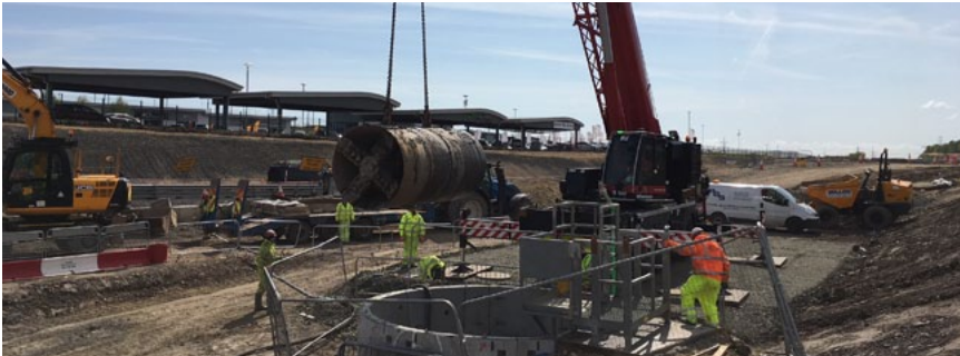
The tunneling machine is lowered into the shaft
