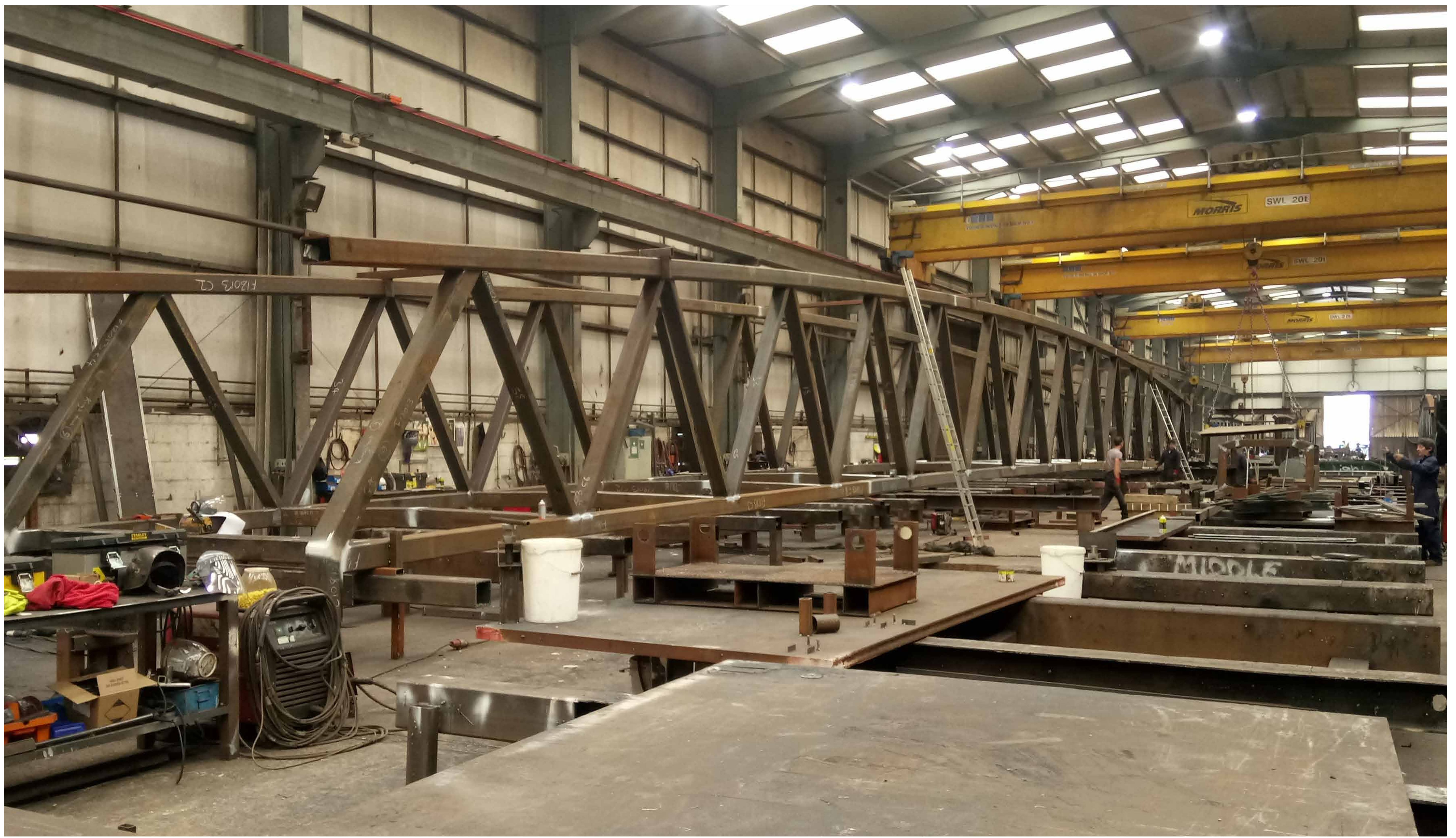
Kingsford Street Bridge being fabricated in Hythe
